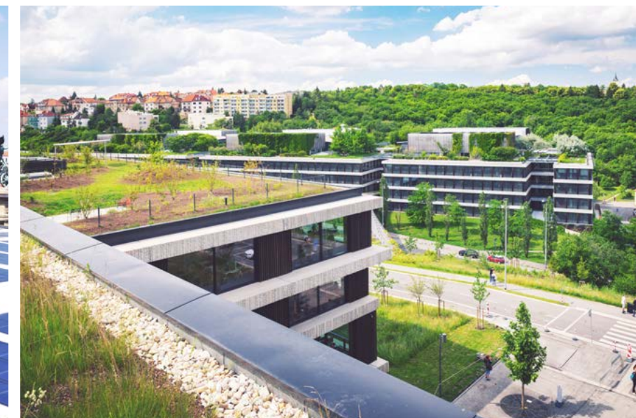
The building of headquarters of bank ČSOB in Radlice is an example of sustainable approach. The heating and cooling using an extensive system of heat pumps is especially unique. The building does not need a classic boiler room. Moreover, the complex efficiently uses rainwater, and thus contributes to savings of drinking water. PHOTO: NADACE PARTNERSTVÍ / VOJTA HEROUT
