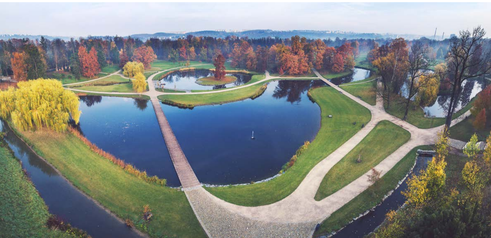
Restoration of the water system of Prague's Stromovka Royal Game Reserve, which was part of the complex revitalization of this popular landscape park, created a pleasant environment. PHOTO: LUBOMÍR STIBUREK
